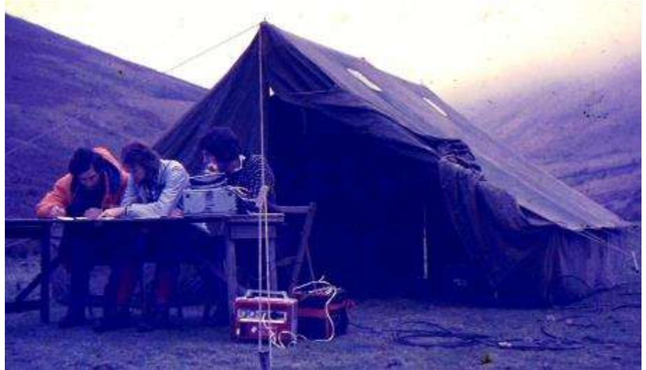
Base set radio on the table with external speaker on top. Small petrol generator which is powering a large lead acid battery which in-turn is the power source for the radio.
