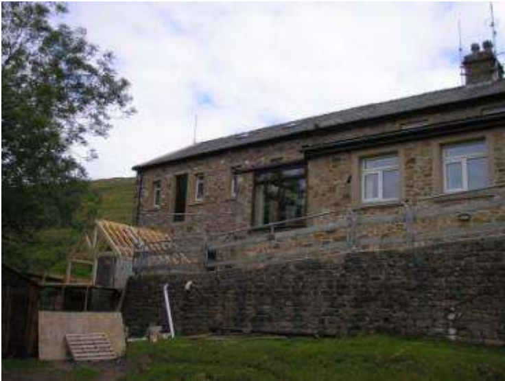
Outside toilet block, uPVC conservatory and railings.
