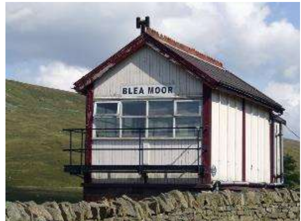
Signal box just before the southern tunnel entrance.
