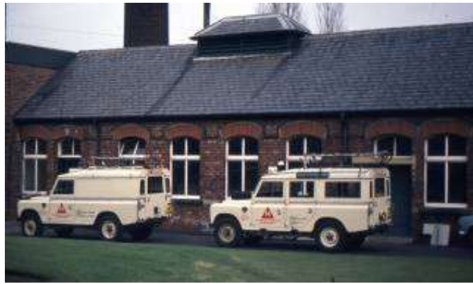
Deepdale Isolation Hospital
